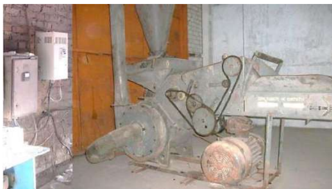
Fig.1. General view of controlling an asynchronous motor of a universal fodder shredder using a frequency converter
